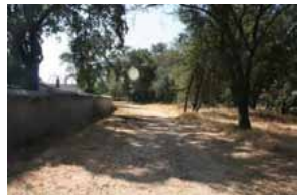
Floodwall along east side of Linda Creek, looking south
