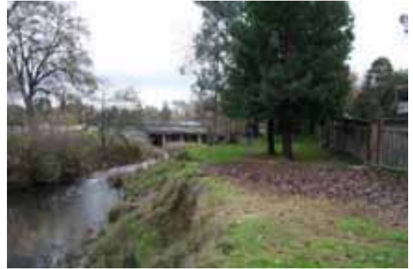
Existing Rocky Ridge Drive box culverts, looking east
