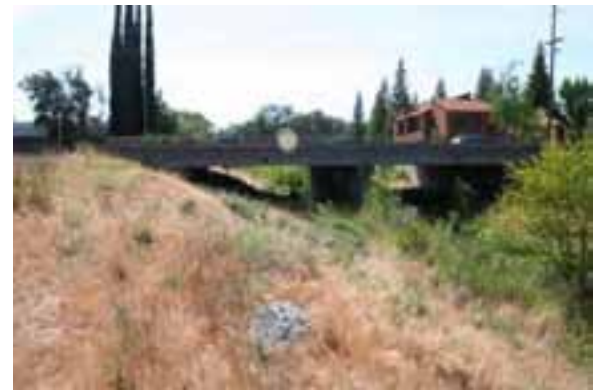
Existing Sunrise Avenue Bridge over Linda Creek (Crossing C), looking west
