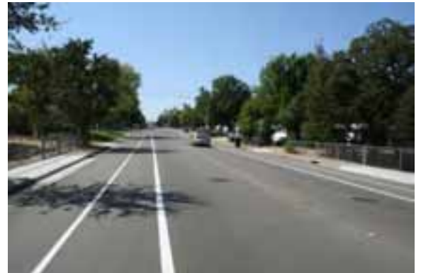
Linda Creek at Champion Oaks Drive; note recently installed bike lanes
