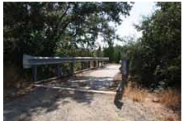
Existing rail car maintenance bridge (Crossing 22) over Strap Creek
