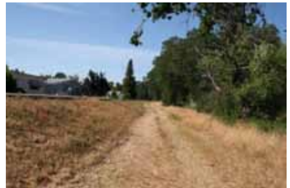
Existing maintenance road and floodwall along west side of Linda Creek, looking north
