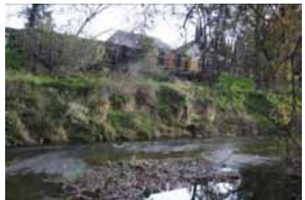
Steep banks, narrow right-of-way and storm sewer manholes along west bank of Dry Creek
